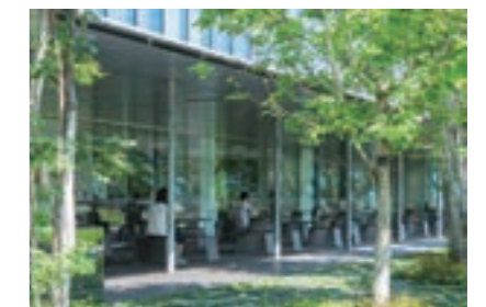
Rooftop Greening (Photo:Waseda Arena, by Shinkenchiku-sha) *Awarded the Minister of Land, Infrastructure, Transport and Tourism Prize of the Organization for Landscape and Urban Green Infrastructure [IBIDEN GREENTEC CO., LTD.]
