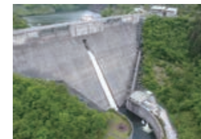
Low Head Hydro Power System [IBIDEN ENGINEERING CO., LTD.]
