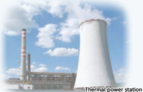
Thermal power station
