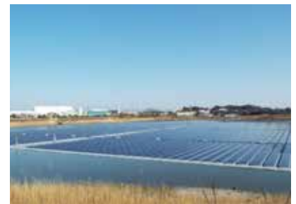
Water floating solar power generation plant at the closed lumberyard parking site of the Kinuura Plan
