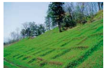
Slope constructed using the GT frame®
