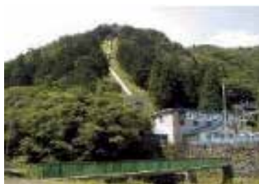
Kawakami Power Plant (Updated in 2014) Power output: 4,400kW
