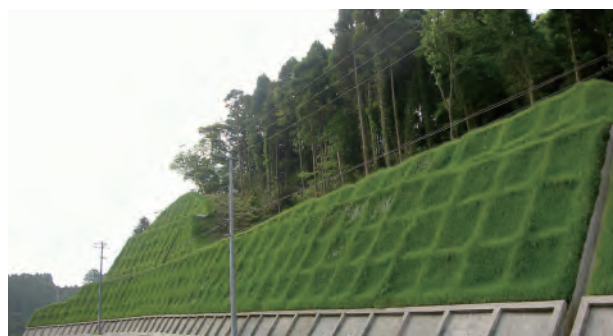
Slope constructed using the GT frame®
