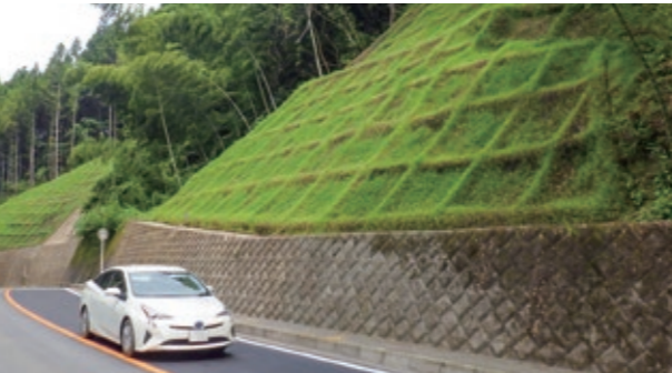
Slope constructed using the GT frame®
