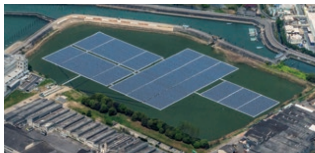
Water floating solar power generation plant (Certificated output:1.99MW)
