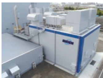
Gas engine cogeneration system
