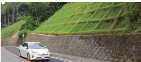
Slope constructed using the GT frame®
