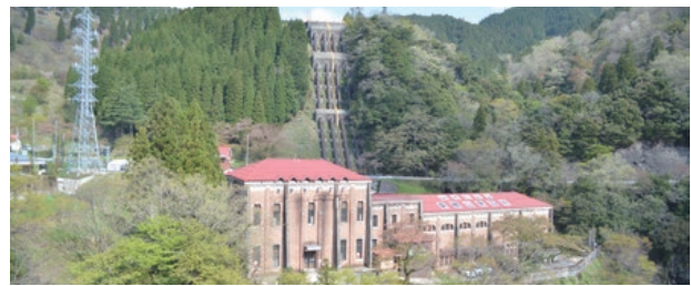
Higashi-Yokoyama Power Plant
