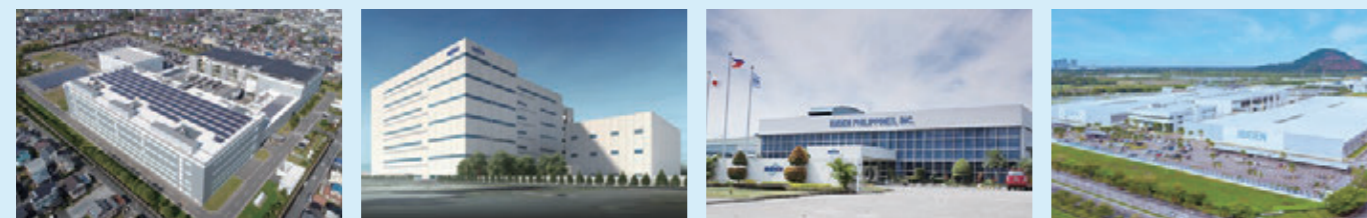
Ogaki Central Plant | Gama Plant ※under renovation | IBIDEN Philippines, Inc | IBIDEN Electronics Malaysia SDN. BHD.
