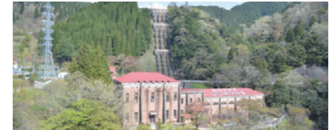
Hydroelectricity (Higashi-Yokoyama Power Plant)
