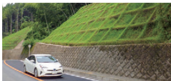
Slope constructed using the GT frame®
