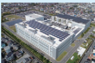
Ogaki Central Plant
