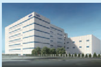
Gama Plant ※under renovation
