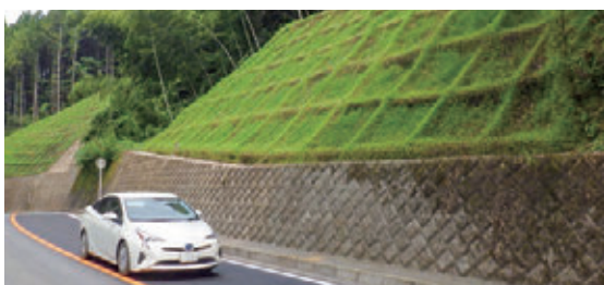
Slope constructed using the GT frame®
