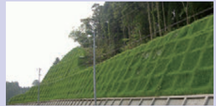
Slope greening for environmental conservation (GT Frame Method®)
