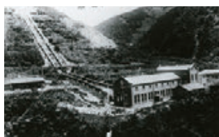
1 Nishi-Yokoyama Power Plant (1916-1963)
