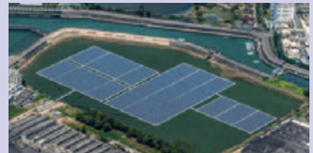
Kinuura Plant Water Floating Solar Power Generation
