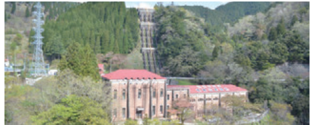
Hydroelectricity (Higashi-Yokoyama Power Plant)
