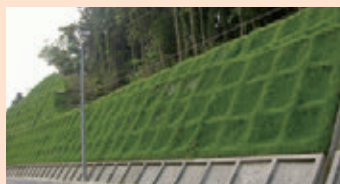
Slope Facing Business (GT frame Method) [IBIDEN GREENTEC CO., LTD.]
