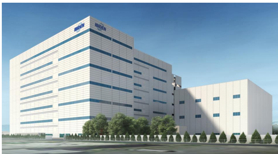
Image of new production building in Gama Plant
