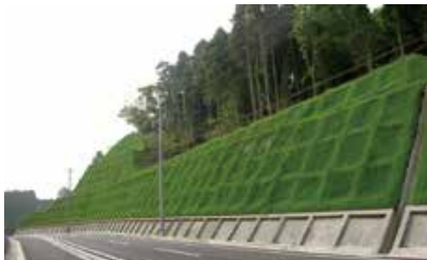
Slope constructed using the GT frame®
