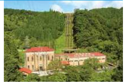
Higashi-Yokoyama power plant
