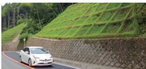
Slope constructed using the GT frame®
