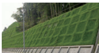
Slope Facing Business (GT frame Method) [IBIDEN GREENTEC CO., LTD.]
